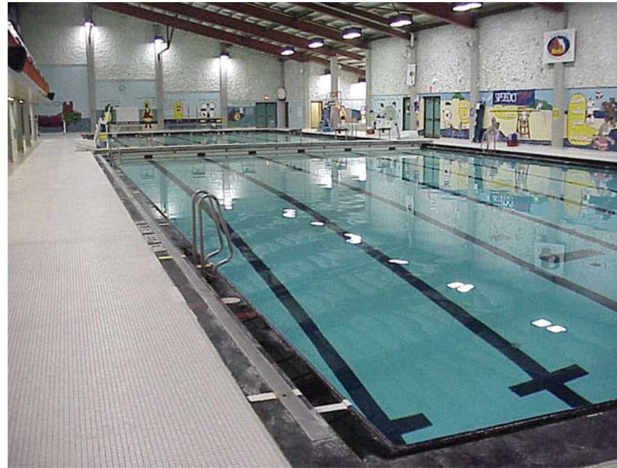
Indoor Pool at the Victoria Road Recreation Centre
