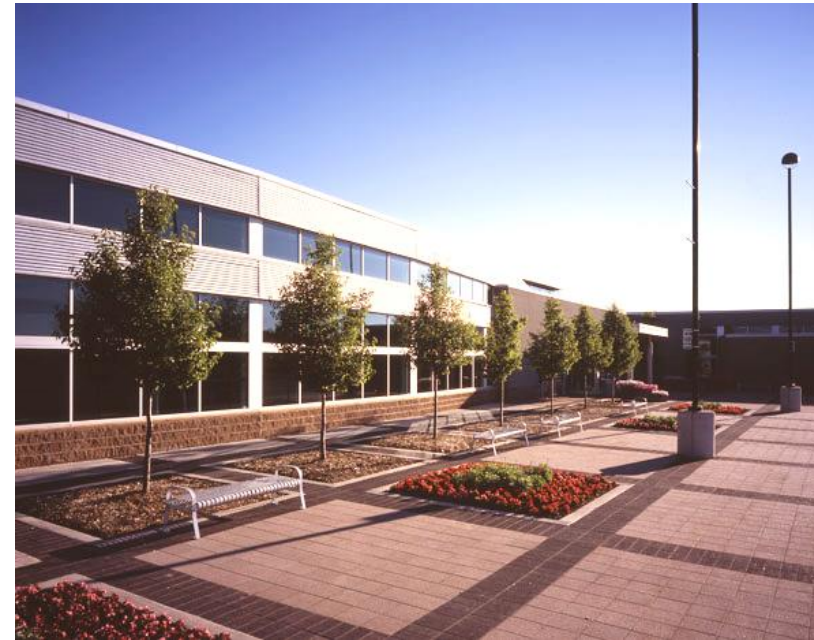
West End Community Centre
